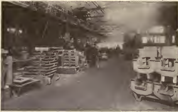
WOOD BLOCK FLOOR IN INDUSTRIAL PLANT
